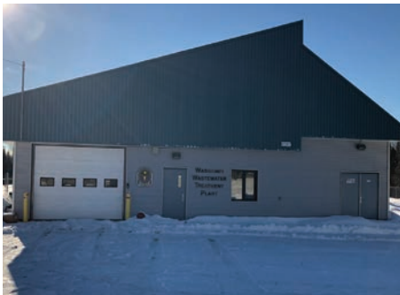
Waste Water Treatment Plant constructed 2012
