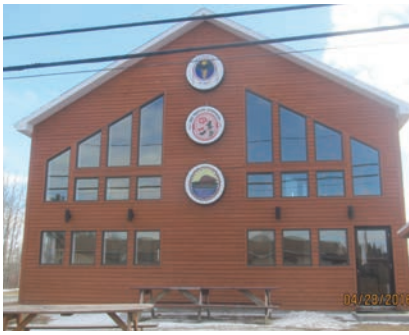
Local Cree Trapper's Association Administration Building 2011
