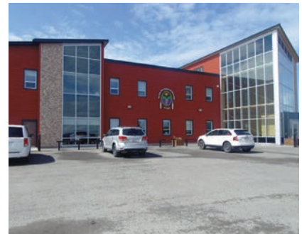
New office administration building, 2009 houses 60 working stations
