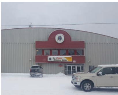
Arena constructed in 1987 currently used for Post Office, Rental Housing Maintenance Office and Storage of Equipment and Material
